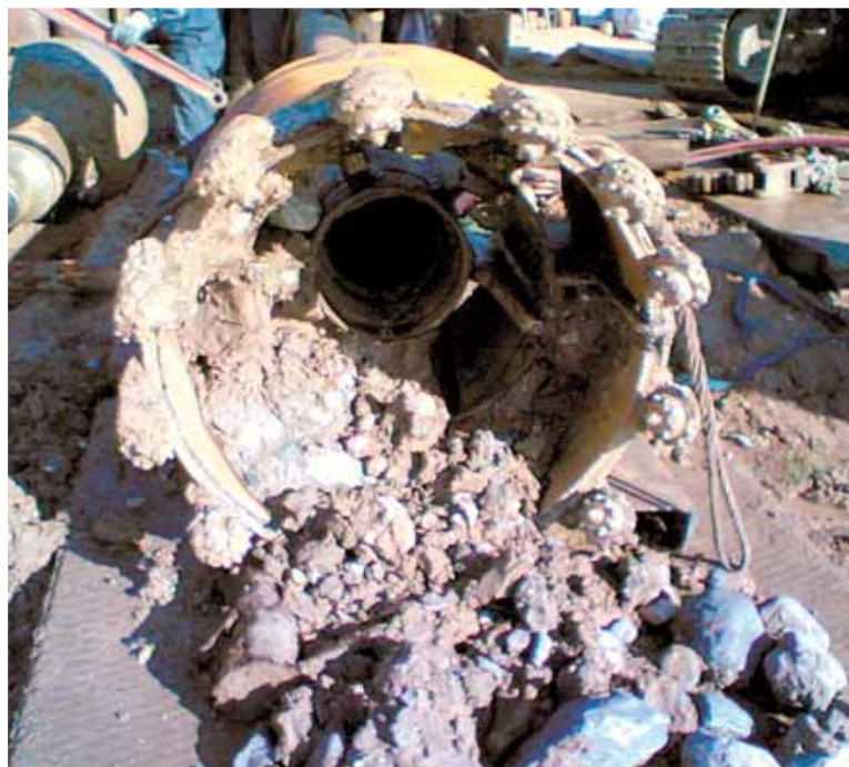
The reamer after demounting, filled with rocks.
